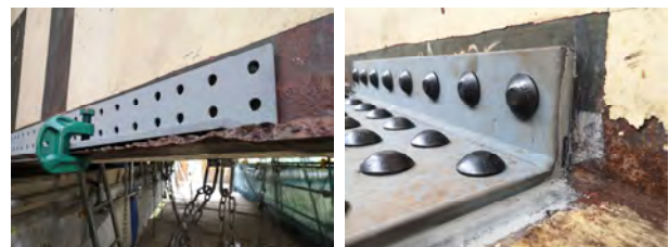
Figure 1. A repair work with epoxy putty and high-strength bolts in Japan
